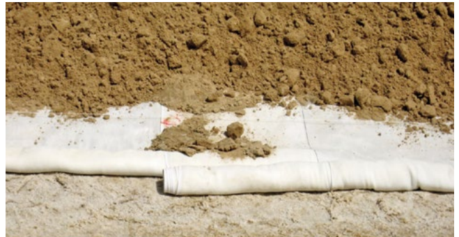
Overlapping sheets with soil cover
