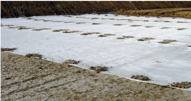
Ballasted / overlapping sheets
