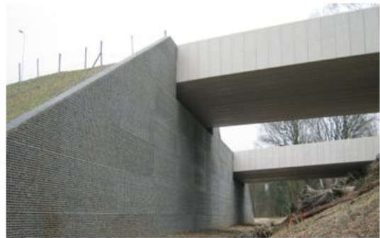
Figure 6. Measurement data of horizontal and vertical deformations during preloading and bridge deck installation as well as pictures of the preloaded retaining wall and finished abutment with installed bridge deck (van Duijnen et al. [2])
