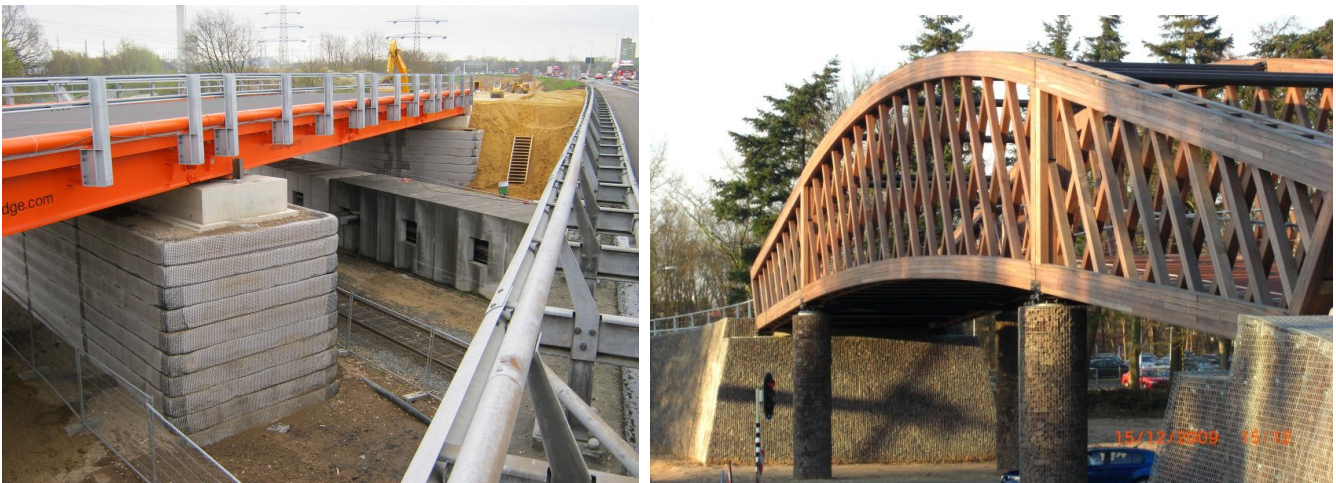
Figure 2. Temporary and permanent bridge abutments in the Netherlands
