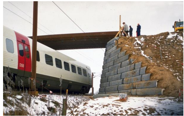
Figure 12 Bridge Abutment Ullerslev in 1991
