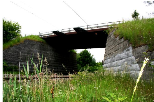
Figure 13 Bridge Abutment Ullerslev in 2013
