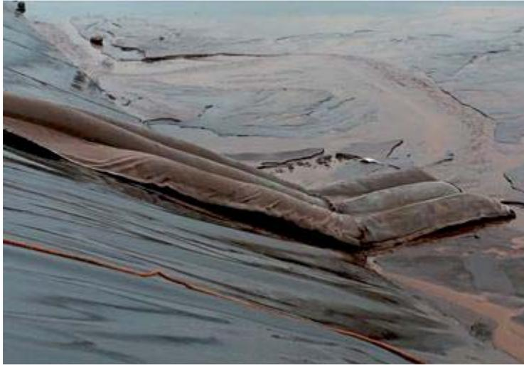
**Figure 7. Installation of geosynthetic protection/ballast layer placed on top of primary geomembrane**
