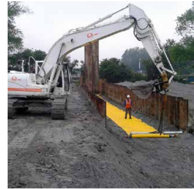
Artère des Hauts de France, DN 900 France: early warning system and excavation protection for gas pipeline with Fortrac PipeGuard geogrid.
