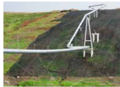
2004 Slope stabilisation, Russia, Baku-Novorossiysk, oil pipeline
