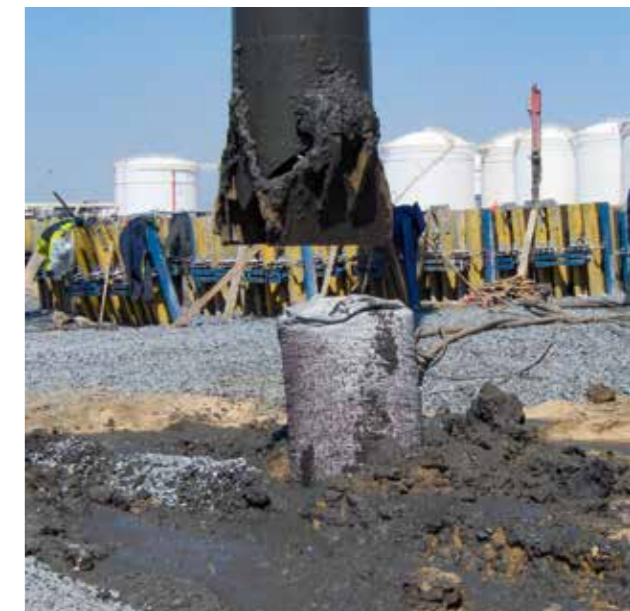
Ground improvement for oil tanks Spain: construction of safe, ductile foundation system in very soft soils with Ringtrac geotextile-encased columns.
