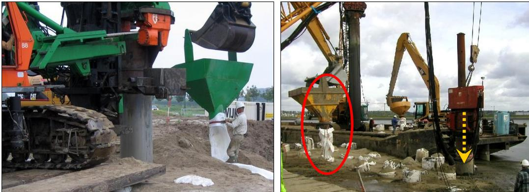
Figure 8: Installation of geotextile encasement (displacement method)
