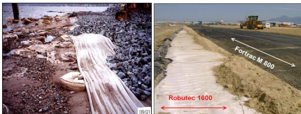
Figure 6: Example of horizontal geosynthetic reinforcement on top of already covered GECs for heavy loaded sensitive runways (left) and under a land reclamation embankment (GECs still visible) (right)
