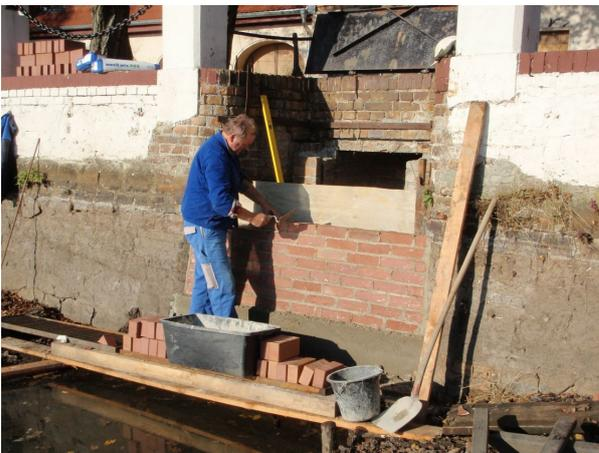
**Fig 5.** Shutting down the old outlet
