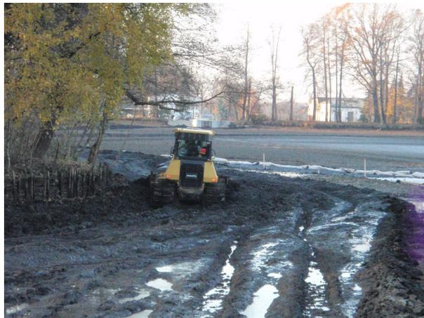
Fig 8. Mass removal of sludge with bulldozer
