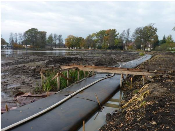
**Fig 13.** Tubes during filling process and new fishing spots still under construction
