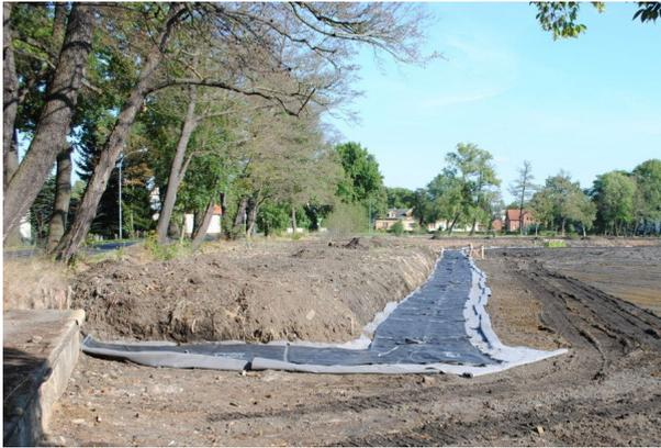
**Fig 12.** Placed non-woven and tubes in construction phase 2 before start of filling process
